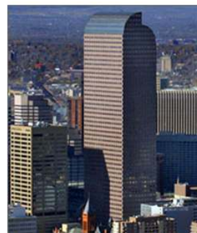
The Fitzmartin Consulting retrofit project involves renovating one floor of the five-floor HRO law offices in the Wells Fargo Center in downtown Denver, Colorado. Photo courtesy of Downtown
