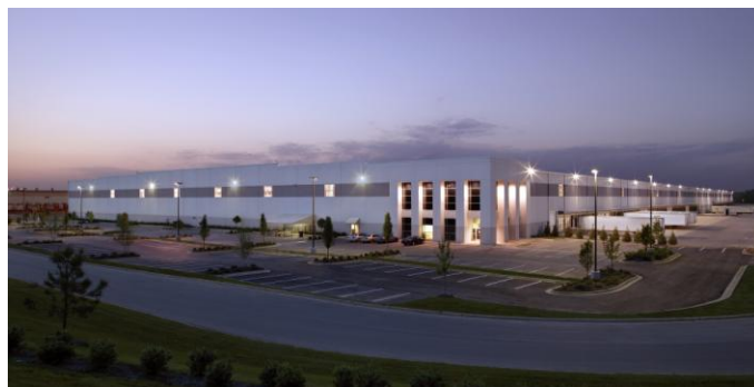
The ProLogis Commercial Building Partnerships retrofit—a simple lighting retrofit on this 800,000 square foot Sears warehouse in northern Mississippi—will save about 30% of the energy the building previously used. Photo courtesy of ProLogis
