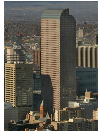
The Fitzmartin Consulting retrofit project involves renovating one floor of the five-floor HRO law offices in the Wells Fargo Center in downtown Denver, Colorado. Photo courtesy of Downtown Denver Partnership
